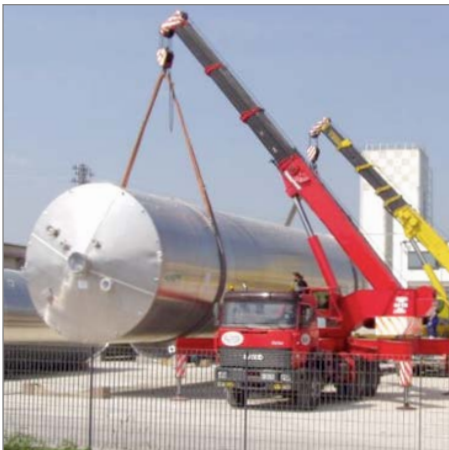
Monolithic silo are shipped with flat rack and they required minimum assembly operations on site
