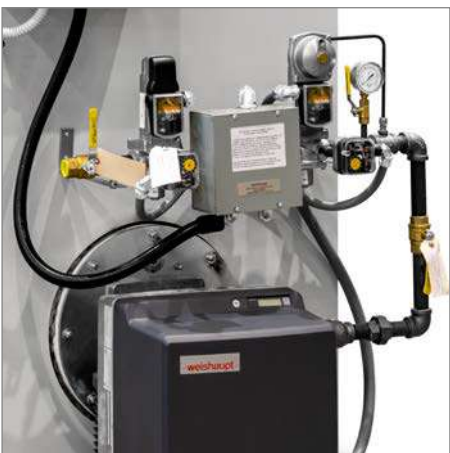
Complete set of pressure switches to check: minimum and maximum process air pressure, minimum gas pressure and burner ventilation
